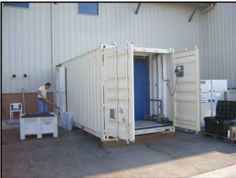
The system is mounted inside a 20 foot intermodal shipping container. This allows the system to be delivered complete with a minimum of site preparation. In this application, the system was simply located outside the winery and installed with no disruption to winery production schedule.
