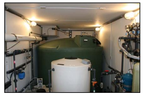
Each system includes an 1800 gallon storage tank for the finished product (the large green tank in the background). The white cylindrical tank in the foreground holds UF filtrate and feeds the RO unit. The rectangular tank near the ceiling in the background hold RO permeate which is used to automatically flush the RO membrane elements upon shutdown of the system.
