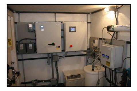
Each system is equipped with a state-of-the-art control system utilizing electronic sensors for flow and pressure monitoring. All control functions are available from a single touch-screen operator interface. The container is insulated with 2 1/2" of rigid foam insulation covered with a 1/16" thick plastic barrier. The insulation is designed for use in wet industrial environments.
