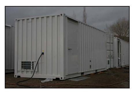
Each system is totally self-contained inside a 20 foot intermodal shipping container. Each container is insulated and equipped with an air conditioner to provide climate control. The system operates from a single 460 volt AC power source.
