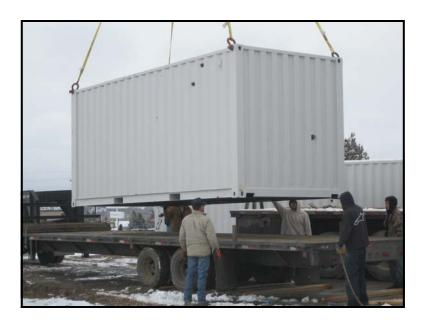
The system is mounted inside a 20 foot intermodal shipping container. It is totally self-contained and equipped with heater to accommodate the cold winter climate of Colorado. The system operates from a single 460 volt AC power source. The portability of this system allows it to be easily moved as the location of the work camp changes.
