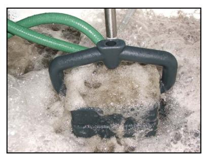
The heart of the MBR system is the submerged membrane modules which separate the suspended solids from the mixed liquor. The ultrafilter membranes reject solids greater than 0.01 micron in size thus generating effluent of superior quality. This photo illustrates the air used to keep the membrane modules clean during operation.
