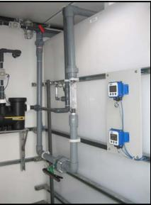
This system is equipped with a state-of-the-art control system utilizing electronic sensors for flow and pressure monitoring. All control functions are available from a single touch-screen operator interface. The container is insulated with 2 1/2" of rigid foam insulation covered with a 1/16" thick plastic barrier. The insulation is designed for use in wet industrial environments.
