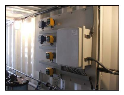
The treatment system is equipped with a state-of-the-art monitoring and control system and a full complement of electronic sensors. Each train is controlled by its own local PLC with a touch screen color operator interface screen. Each local PLC is networked via industrial Ethernet to a single supervisory controller. The supervisory controller is equipped with a cellular network gateway that allows the entire system to be monitored and controlled remotely.
