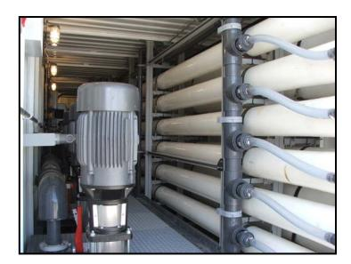
The system is comprised of four separate 500,000 gallon per day trains. Each train is housed in a 40 ft intermodal shipping container. Each train is fed by three vertical centrifugal high pressure pumps, each representing 50% of full capacity. The pumps are piped in parallel thus allowing 50% standby pumping capacity.
