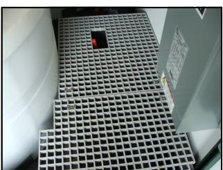
A raised floor inside the containers provides a clean, uncluttered work area.
