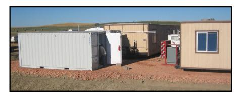
RODI's containerized membrane bioreactor systems have proven effective at treating the high strength waste from portable toiler facilities at remote work locations. Typical performance data are shown below.
