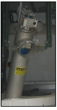
The RODI treatment systems have many other features normally seen in larger treatment plants. Here is shown a small inlet screen designed to remove trash and larger objects that might affect the performance of the system.
