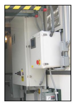
The systems are equipped with a state-of -the-art monitoring and control system. All normal treatment functions are completely automated. Data is automatically logged by the control system to facilitate analysis of the system performance.
