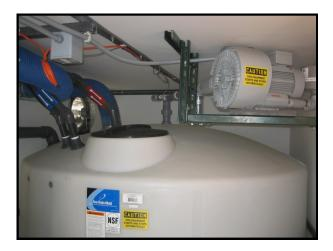
RODI's containerized membrane bioreactor systems are aerobic systems that utilize atmospheric oxygen to allow bacteria to digest the organic waste in the sewage. A high performance membrane then separates the suspended biomass from the treated water. This allows RODI's system to produce treated effluent of highest quality.
