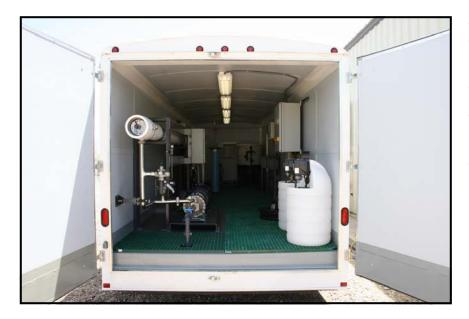
This is the rear of the trailer with the cargo doors open. Note the raised floor which allows piping and conduit to be hidden and protected. This also makes for a very clean installation inside the trailer. The RO pressure vessel and high pressure pump can be seen on the left. The chemical injection systems for pH control and scale inhibitor are on the right.
