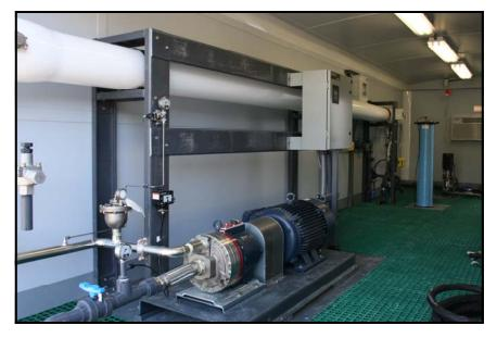
This application utilized a Wanner Hydracell positive displacement pump. The Hydracell pump has proven to be durable and is easy to rebuild when necessary. The Hydracell does need to be equipped with a pulsation dampener which can be seen on the top of the pump discharge piping.
