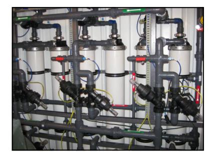
The final pretreatment step before the RO trains is a capillary fiber UF system. This was required due to the fact that the source of the feed water was a harbor subject to high turbidity. The UF service, backflush, and chemically enhanced backflush (CEB) steps were all completely automated.
