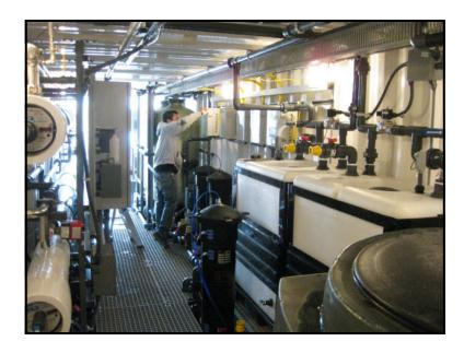
The system is totally contained in a 40 foot intermodal shipping container. Efficient use of the space inside the container was critical due to the complexity of the treatment system. The system operates from a single 460 volt AC power source.
