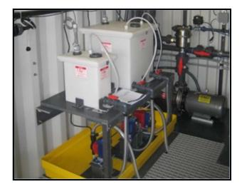
Chemical injection systems are provided for chemically enhanced backflush as well as normal on-going chemical disinfection (chlorination) of the product water produced by the system.
