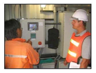
The system is equipped with a state-of-the-art monitoring and control system. All normal treatment steps, including service, backflush, and chemically enhanced backflush (CEB), are completely automated. Data is automatically logged by the control system to facilitate analysis of the system performance.
