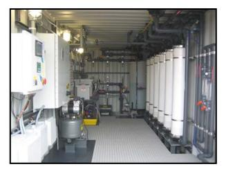
The system is totally contained in a 20 foot intermodal shipping container. All components of the treatment system are mounted inside the container. Hollow fiber microfiltration was chosen for this application due to the high turbidity (300 NTU) of the feed water.
