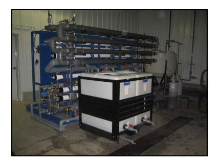
The system is mounted on an epoxy coated steel skid. The tubular UF, both RO units, and controls are all contained on the skid. The system also comprises two RO feed tanks and a cone bottom recirculation tank for the UF unit. Treatment capacity of the system is 12,000 gallons per day with recovery approaching 85%.
