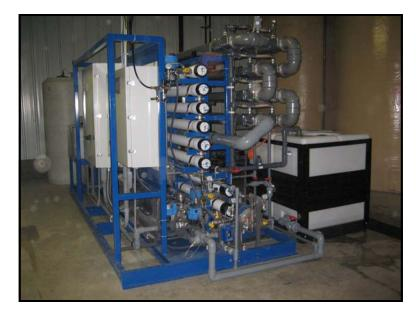
Dissolved solids concentration of the feed water can exceed 5,000 ppm with the concentration of the final RO reject approaching 35,000 ppm. Thus the secondary RO unit is equipped with seawater vessels and membrane elements.
