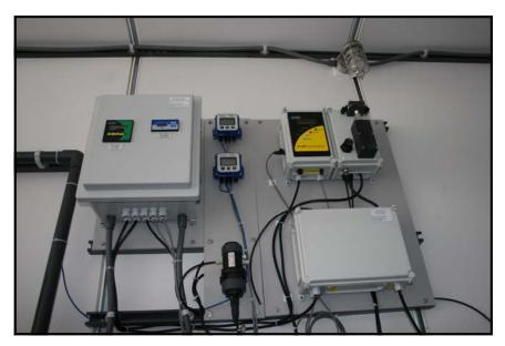
The system is equipped with a full complement of monitoring equipment. This includes turbidity as well as silt density index utilizing RODI's proprietary EZ SDI<sup>TM</sup> automatic silt density index monitor.
