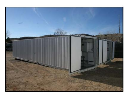
The system is totally self-contained inside a 40 foot intermodal shipping container. The container is insulated and equipped with an air conditioner to provide climate control. The system operates from a single 400 volt 50 Hz AC power source.
