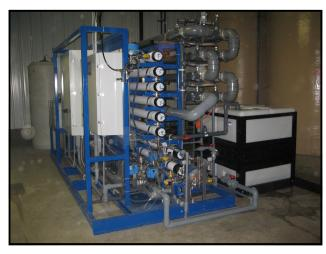
**Pressure Vessels** — All pressure vessels are PVC, stainless steel, or filament wound using fiberglass roving and sealed with an epoxy resin. This results in a corrosion-proof system that will last for years with minimal maintenance.
