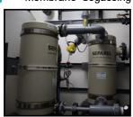
Membrane Clean-in-Place System — Larger systems may include an integral clean-in-place (CIP) system for routine chemical cleaning of the RO membrane elements. This eliminates the need to remove the elements for cleaning off site
